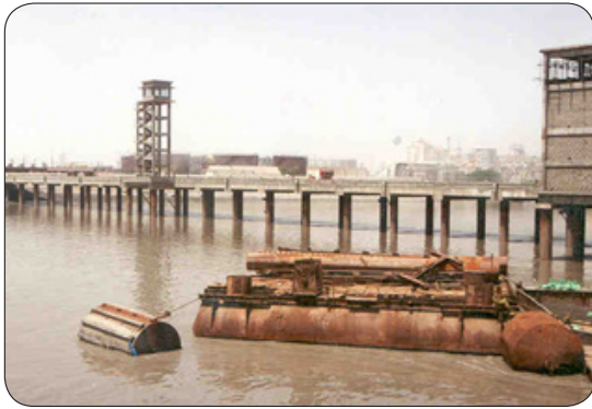
Kandla Oil Jetty
