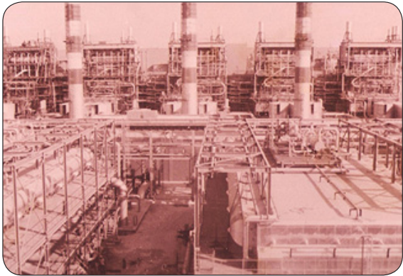
Tripoli West Thermal Power Station
