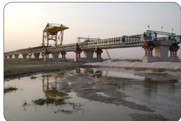
Camel Gantry for Segment Launching
