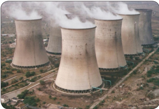
Raichur Cooling Towers
