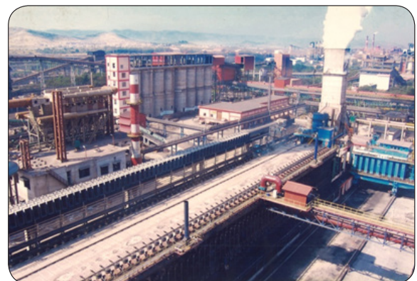
Vijay Nagar Steel Plant
