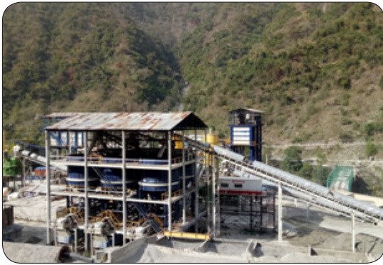
Temperature Controlled Concrete Production
