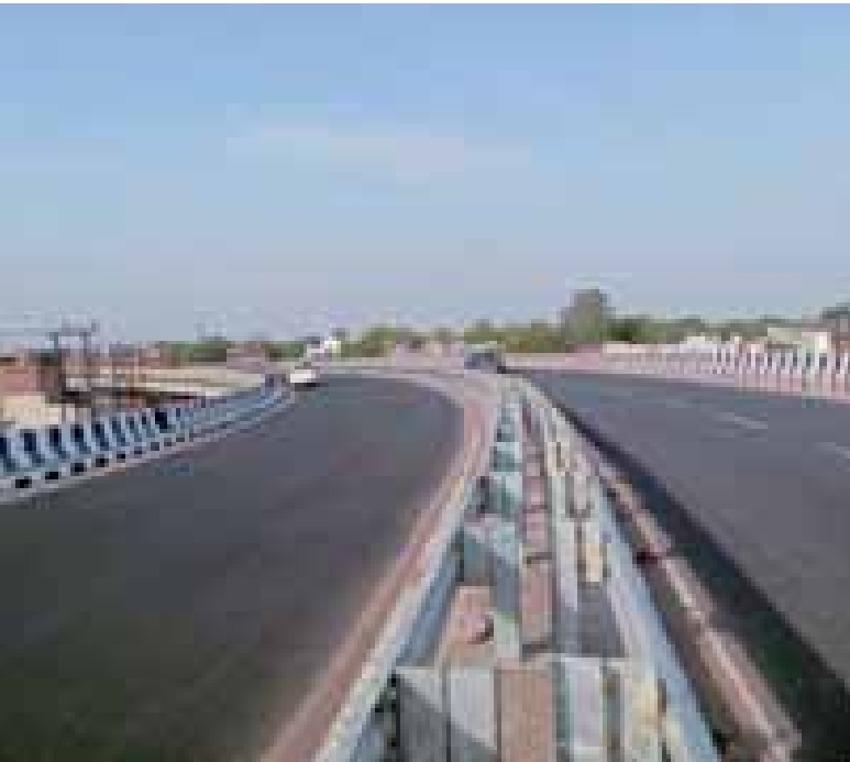
Ganga Bridge, Kanpur
