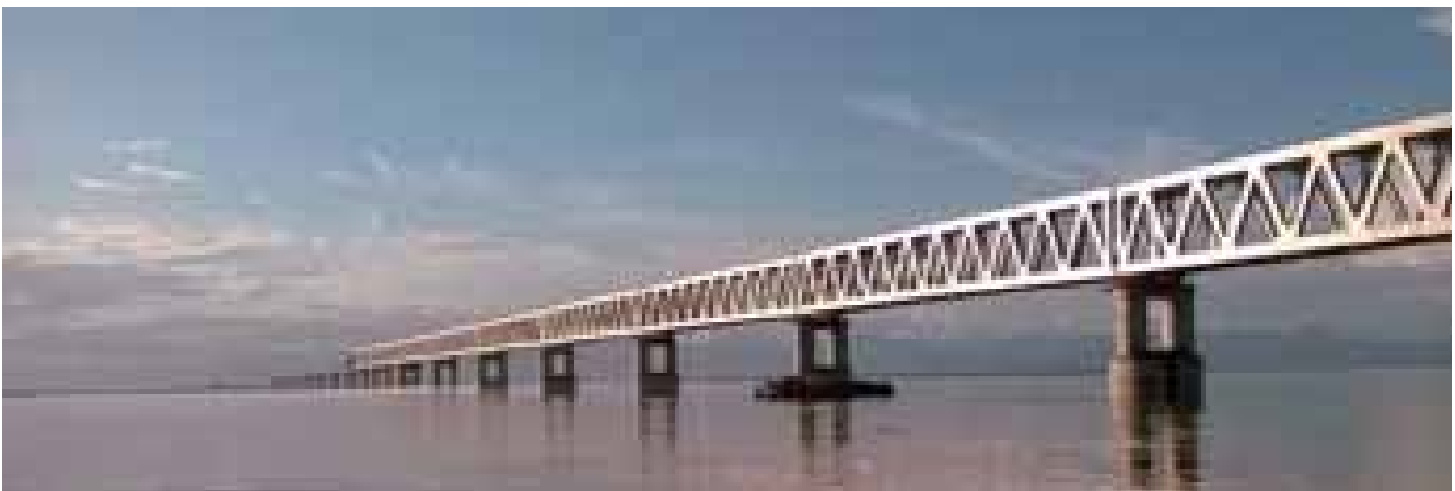
Bogibeel Bridge, Assam
