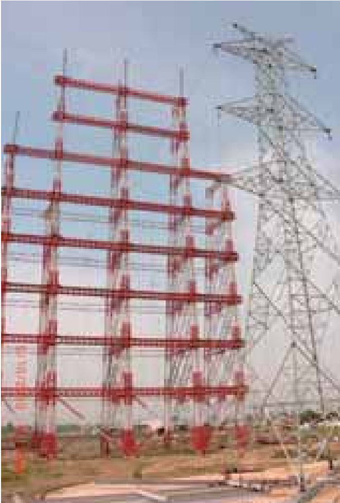
765 KV Dc Type Testing Tower, Deoli, Maharashtra
