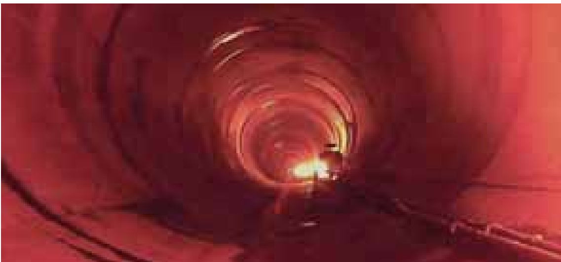
Head Race Tunnel , Bhutan
