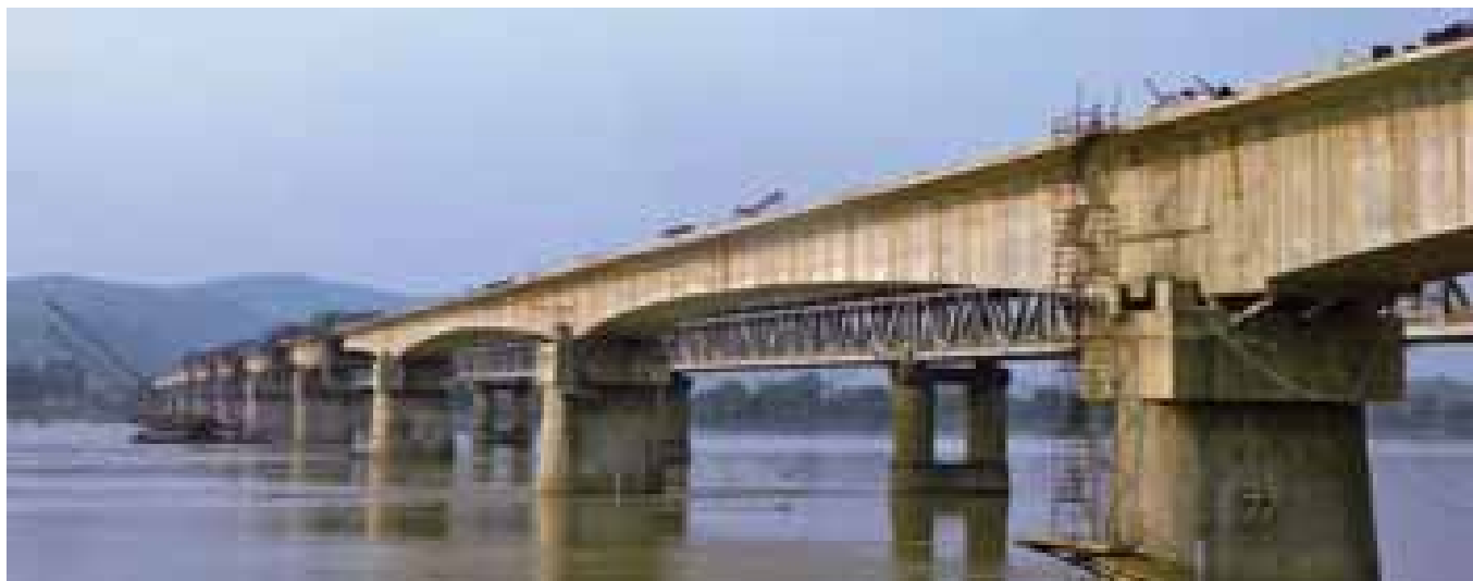
New Brahmaputra Bridge, Guwahati, Assam
