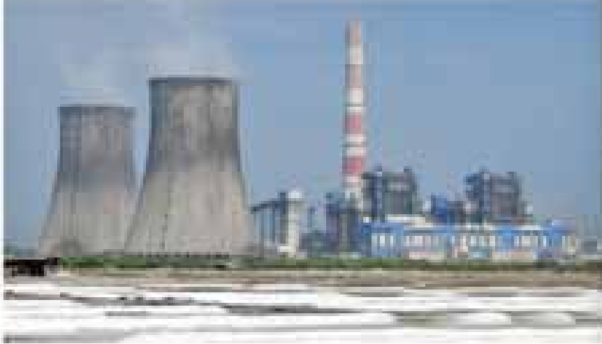
Cooling Towers and Chimneys, Tuticorin
