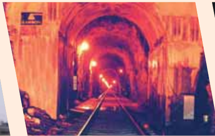
Railway tunnel of seven kilometres for Konkan Railway at Ratnagiri, Maharashtra, in 1995, the longest in Asia at that time
