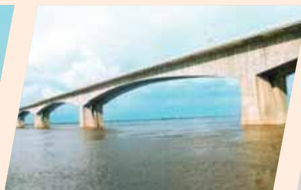
River bridge of six kilometres across the Ganges at Patna, Bihar, in 1982, the longest in India at that time
