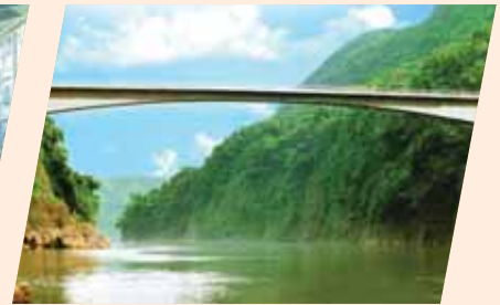
Longest span Cantilever bridge of 140 metres across the river Jadukata, Meghalaya, in 2001
