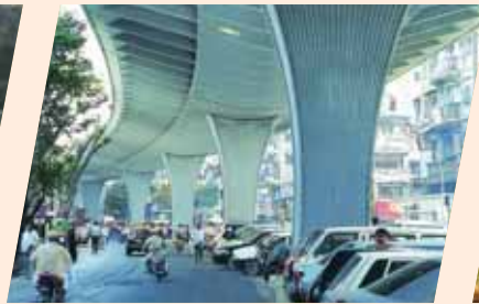
Urban viaduct of two kilometres at J.J. Hospital, Mumbai, in 2002, the longest in India at that time
