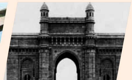
First reinforced piling job in India for construction of the foundation of Gateway of India, Mumbai, Maharashtra, in 1922
