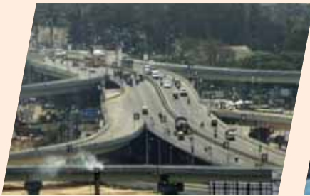
Clove leaf flyover of five kilometres at Hebbal, Bangalore, in 2003, the longest in India at that time
