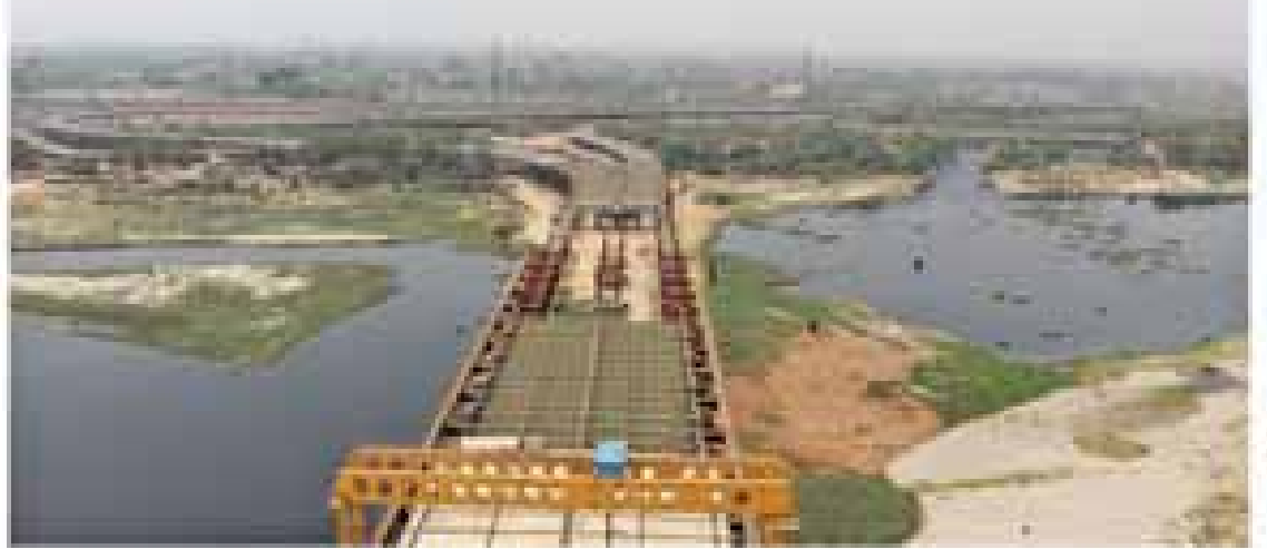
Signature Bridge, New Delhi
