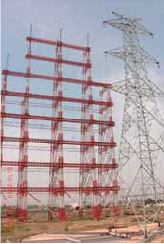
765 KV Dc Type Testing Tower, Deoli, Maharashtra
