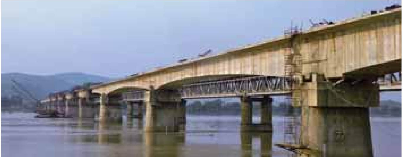
New Brahmaputra Bridge, Guwahati, Assam
