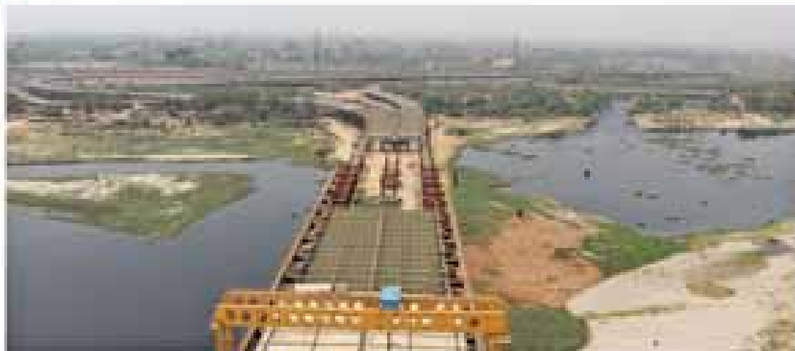
Signature Bridge, New Delhi
