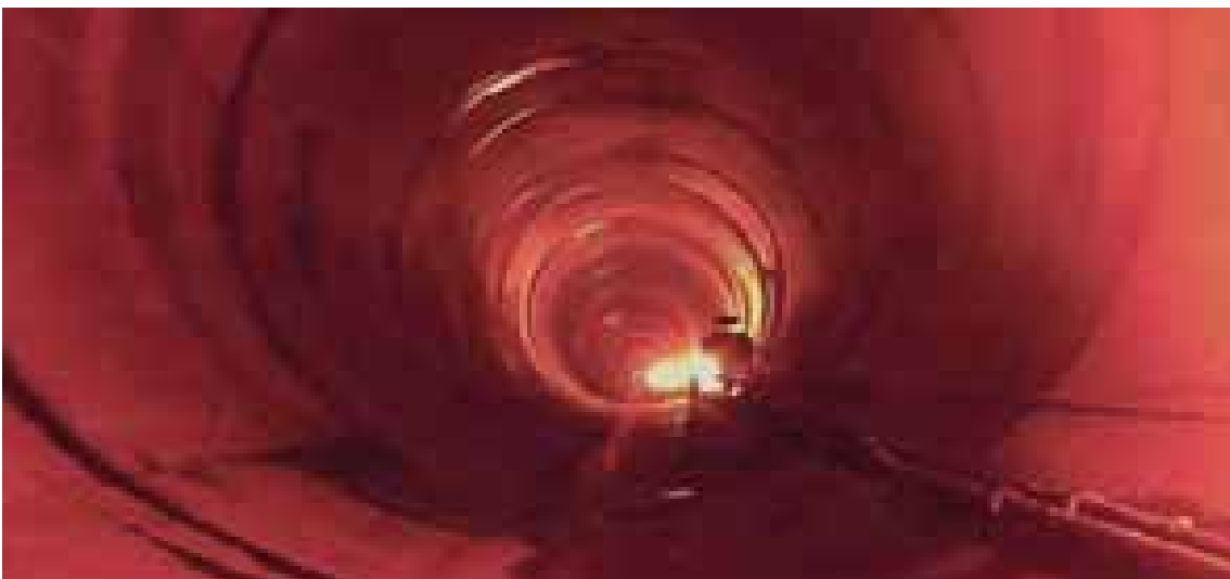
Head Race Tunnel , Bhutan
