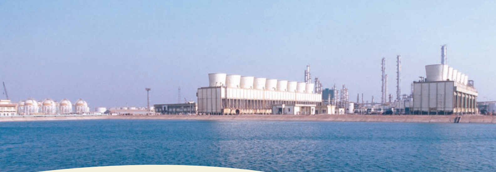
Haldia Cooling Towers
