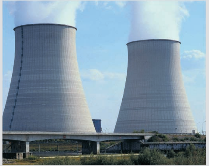
Neyveli cooling Towers
