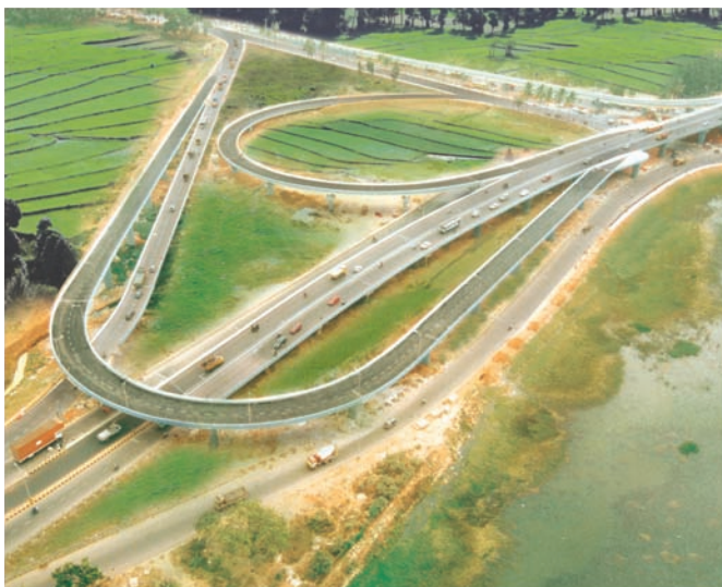
Hebbal Interchange Bridge
