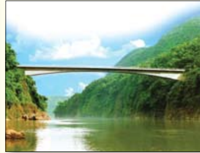
Longest span Cantilever bridge of 140 metres across the river Jadukata, Meghalaya, in 2001
