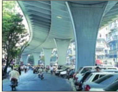
Urban viaduct of two kilometres at J.J. Hospital, Mumbai, in 2002, the longest in India at that time
