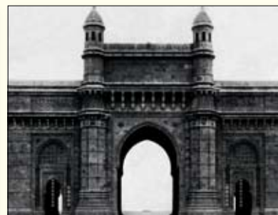
First reinforced piling job in India for construction of the foundation of Gateway of India, Mumbai, Maharashtra, in 1922
