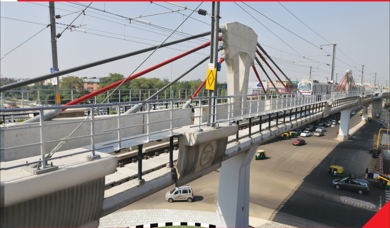
Extradosed Bridge built by Gammon for Delhi Metro
