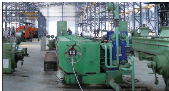
Conductor Factory at Silvassa
