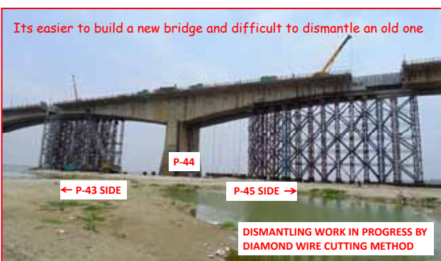
Repairs Works at Old Ganga Bridge, Patna, Bihar
