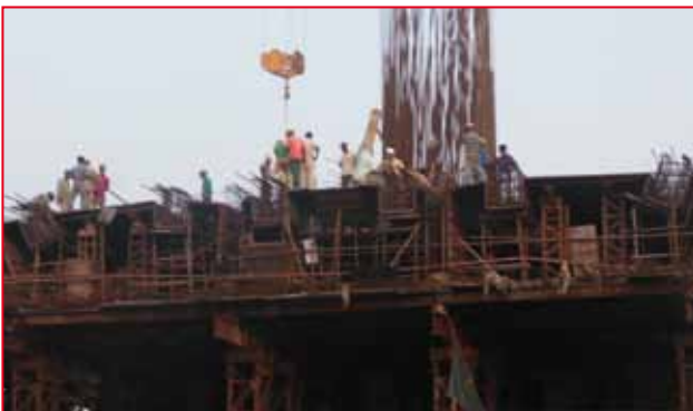
Pylon Pedestal Casting at Surat Cable Stay Bridge, Surat
