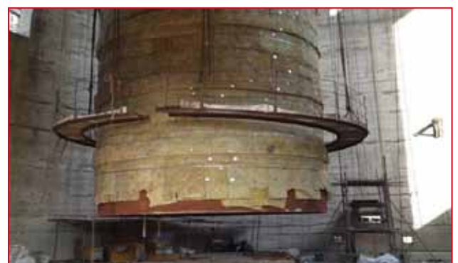
Flue Can Erection for Chimney, Sagardighi, West Bengal
