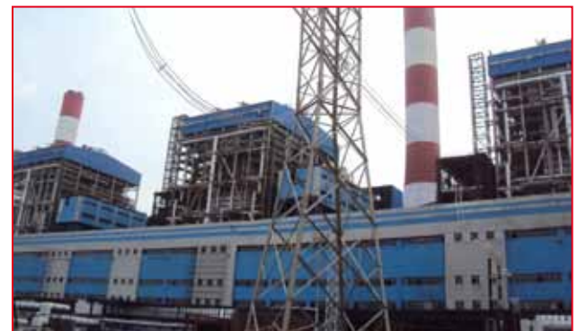
General Civil Works for 3 x 660 MW Power Plant at Sasan, MP
