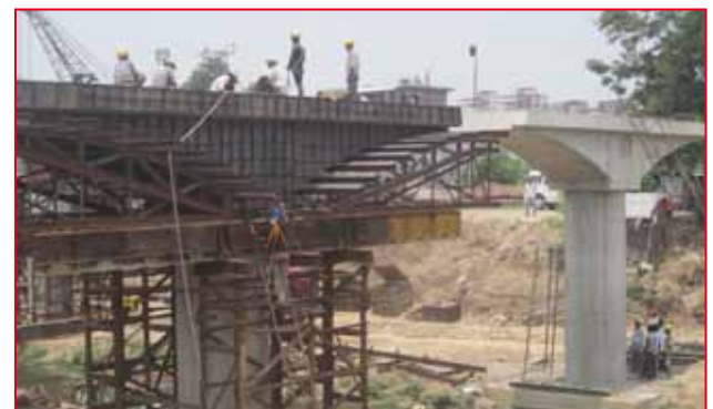
Sub-structure Works at Gangapath Elevated Road, Patna, Bihar
