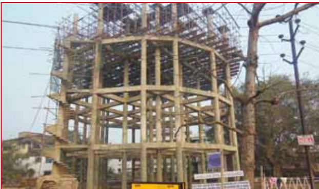
Elevated Water Tank at Patna, Bihar
