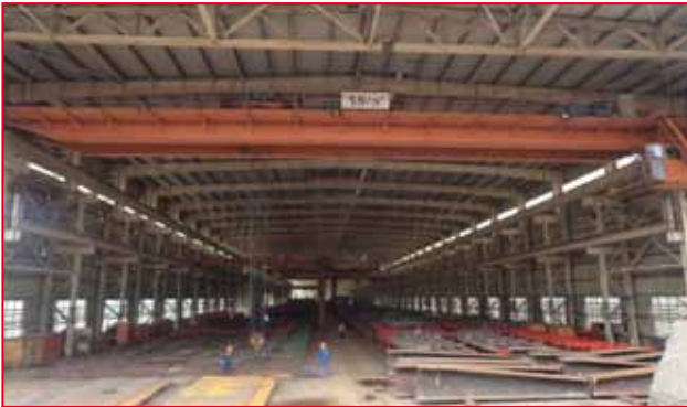
Pylon Fabrication shop in China for Signature Bridge
