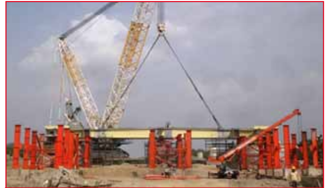
Pylon base erection at Signature Bridge, Delhi
