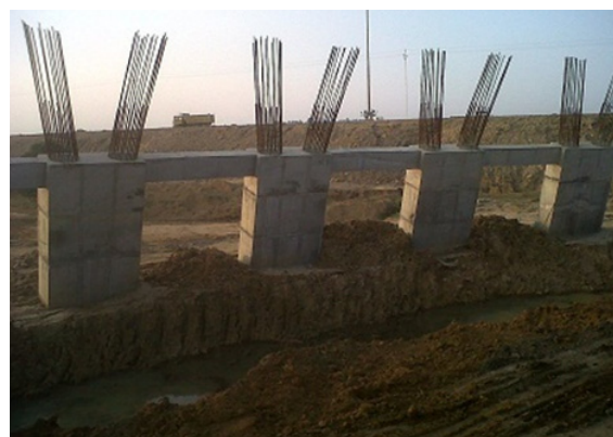
Ring Raft & Pedestals from 15.01.2011 to 25.09.2011
