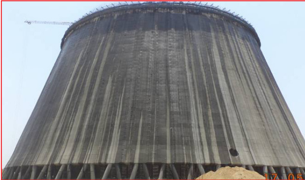
172 m tall Cooling Tower Shell in Progress at Krishnapattanam for Tata Power
