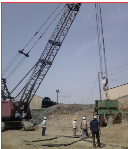
Crawler Crane with Vibro Hammer
