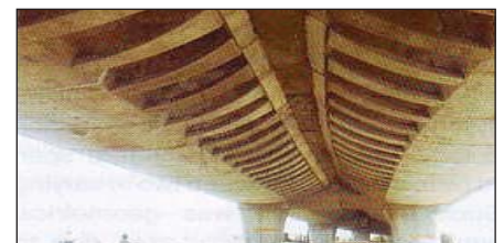
Photo 31: Transition zone-3 - twin boxes (use 12.0 m wide deck) with curtailed arm on one side were joined by cast-in-stitch (of varying width) while other carriageway was made with regular
