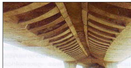
Photo 29: Transition zone-1 - boxes (12.0 wide each) of dual carriage way were joined by cast-in-stitch (of varying width)
