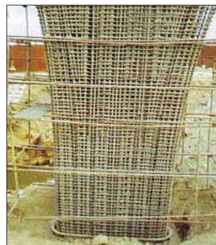
Photo 34 : Reinforcement detail of pier-compatible to requirements of high seismic zones
