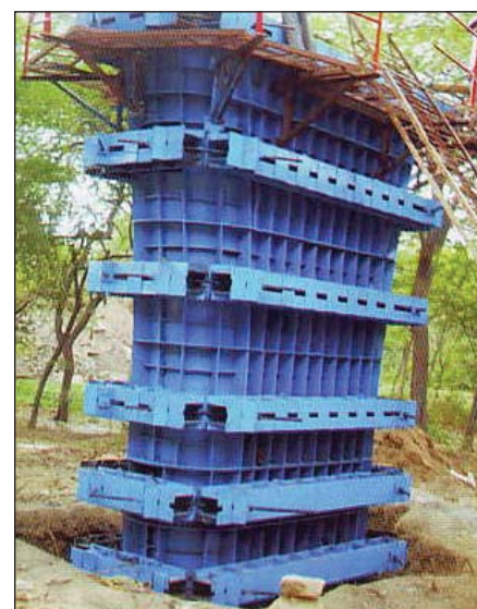
Photo 35 : Shuttering for pier (self compacting concrete is used)
