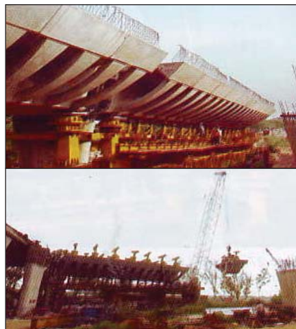
Photo 21 and Photo 22: Ground supported trestles/ staging supporting segments lifted by crane
