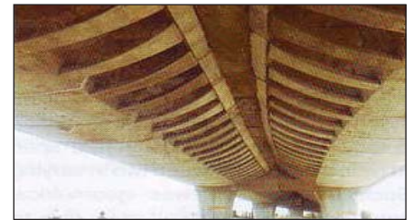
Photo 30: Transition zone-2 - twin boxes (use 10.3 m wide deck) with curtailed arm on one side were joined by cast-in-stitch (of varying width) while other carriageway was made with regular
