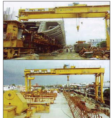
Photo 23 and Photo 24: Ground supported trestles/ staging supporting segments lifted by portal gantry straddling two carriageway width (30 m approx)
