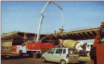
Photo 27 : Self compacting concrete is poured with pumps
