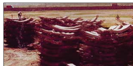
Photo 13: Multiple level of stacking of curved ribs
