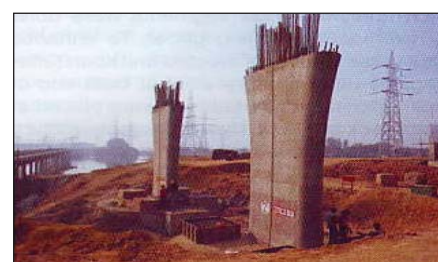
Photo 36 : Intermediate pier of unit (1.2 m thick at top & bottom & 1.0 m thick in center)
