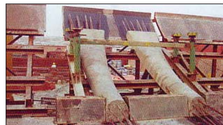
Photo 14: Placement of ribs of segments in long line bed
