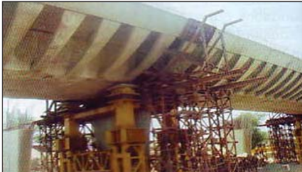
Photo 26 : Staging and precast rib put in position for in-situ connection of superstructure units with pier
