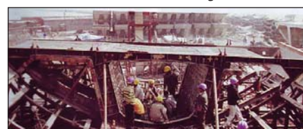
Photo 16: Placement of pre-fabricated reinforcement cage in mould
