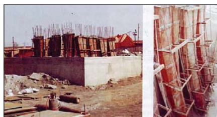
Photo 11: and Photo 12: Tub for casting of curved ribs-base of tub filled with sand to embed projected reinf at the end of curved rib
