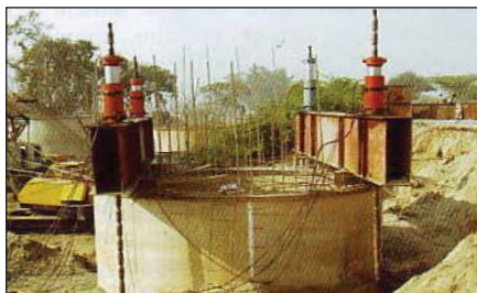
Photo 38 : Jack down method employed for sinking of well
