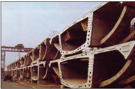
Photo 18 : Multiple tier stacking of precast segment
