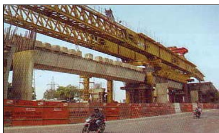
Photo 32 and Photo 33: Erection of unsymmetrical Segments by overhead launching girder
