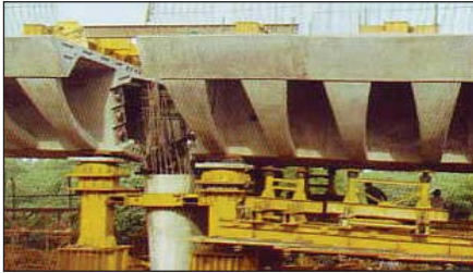
Photo 25 : Erected superstructure rested on end trestles with gap between two units with pier reinforcement projected between two units
