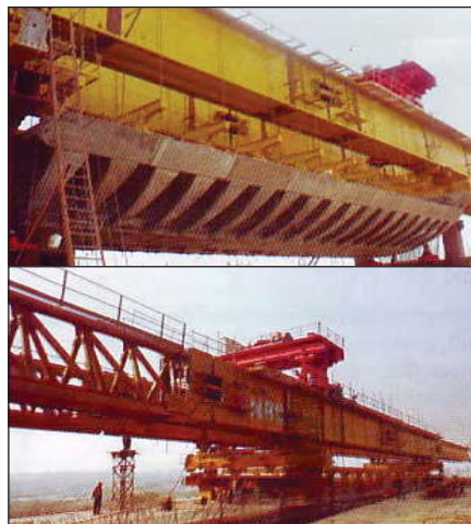
Photo 19 and Photo 20: Precast segments are hung from launching girder
