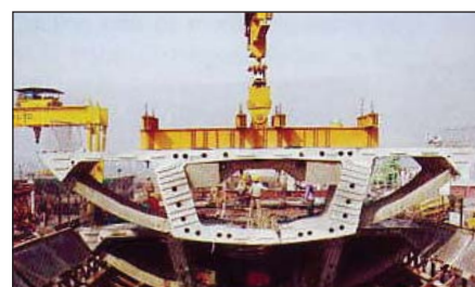
Photo 17: Lifting of segment from bed
