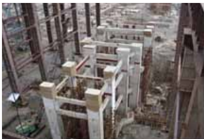
TG Deck Erection Stage
