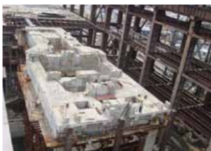
TG Deck after Casting
