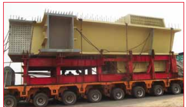
385 t Pylon Base in transit for Signature Bridge, Delhi
