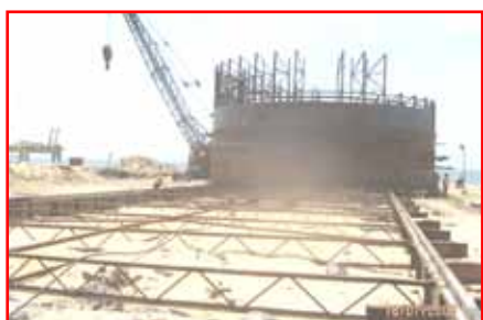
Caisson fabrication above rails
