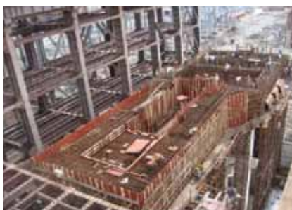
TG Deck Reinforcement & Shuttering
