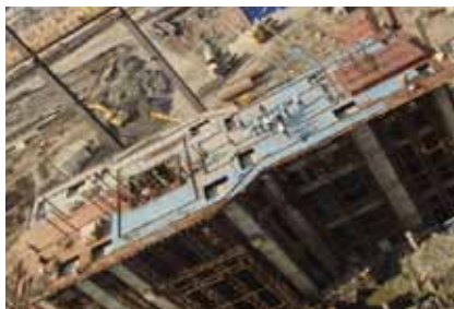
TG Deck Embedded Parts Placement
