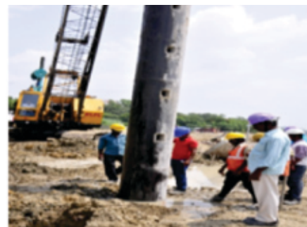
Removing of Stop end tube
