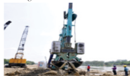
Trenching With Hydraulic Rig
