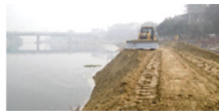
Bund making for Construction of Guide Wall
