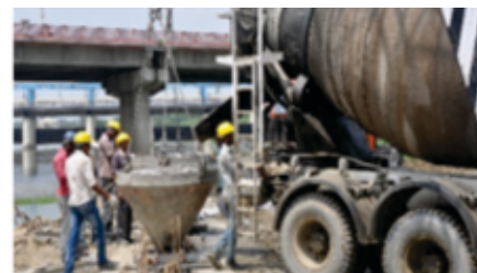
Concreting of D-Wall
