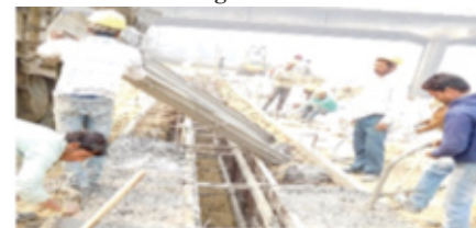
Concreting of Guide Wall
