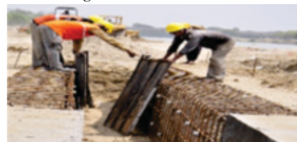
Shuttering for Guide Wall
