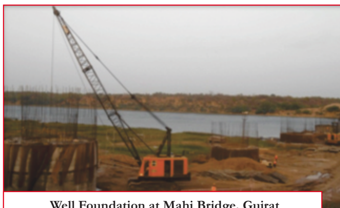
Well Foundation at Mahi Bridge, Gujrat
