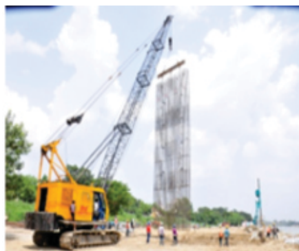
Placing of Reinforcement Cage
