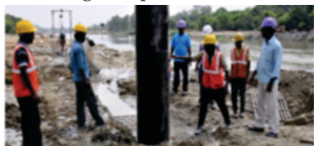
Fixing of Stop End tubes
