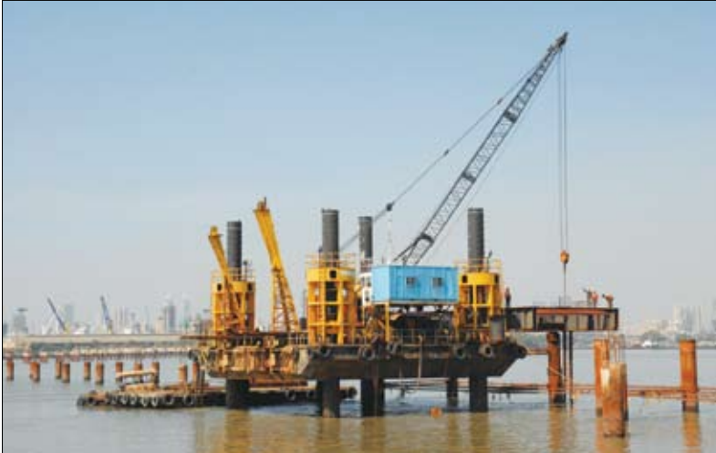
▲ Work in progress at the MbPT
